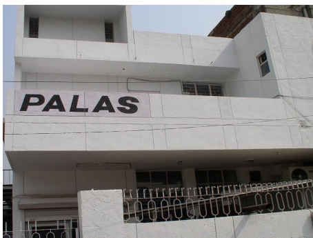
Easily Accessible Location
